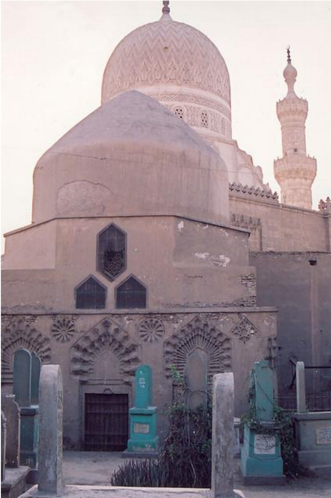
Plate 45: Shrine of the Abbasid Caliphs Image Source: Archnet.
