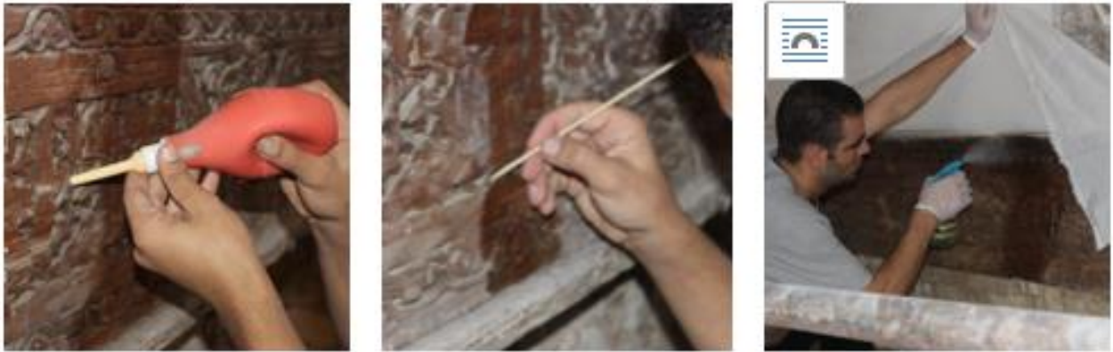
Cleaning, treating with insecticide and dammar.
